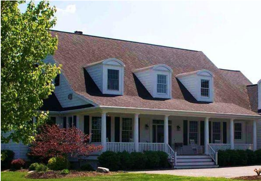
Front porch addition with integrated roofline.
