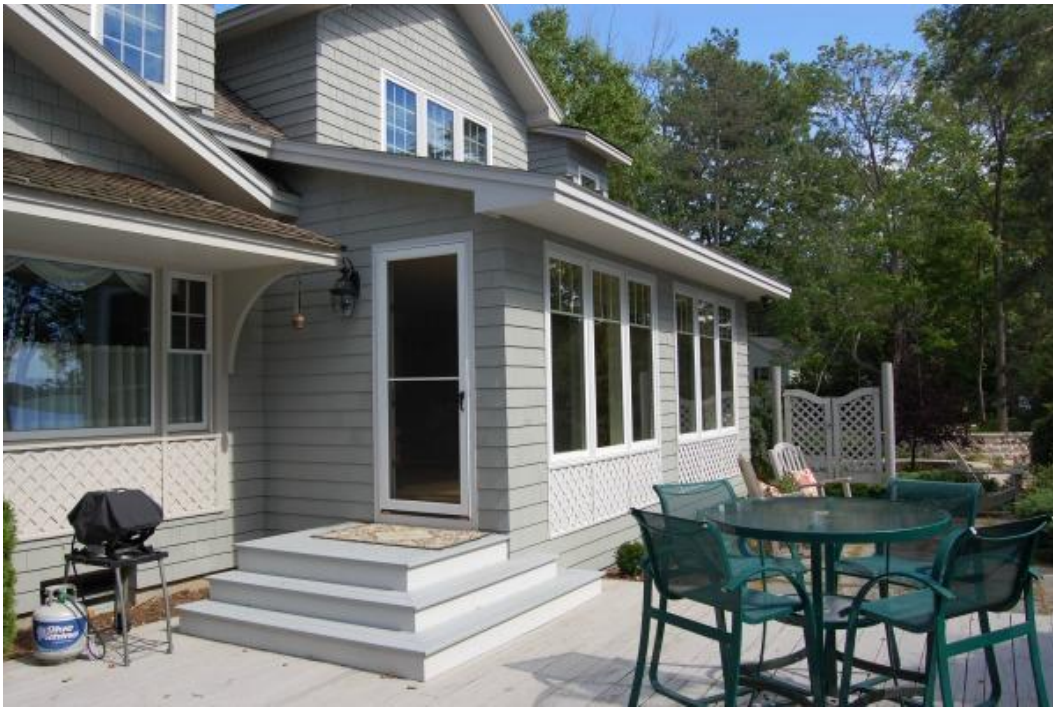
This first floor family room addition blends with the architecture, adds interior space and integrates the home with a cedar deck and yard.
