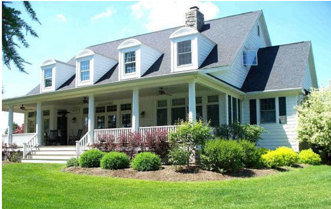
Large, open back porch addition with integrated roofline.
