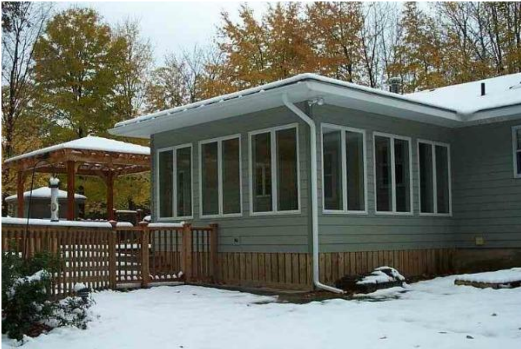
This sunroom addition was built onto the back of a ranch-style home and opens to a deck with a lit gazebo.
