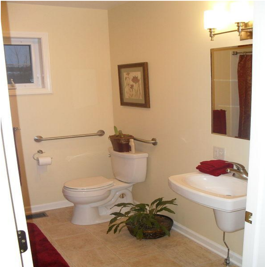
Universal design elements in this master bath include a wall hung sink and grab bars around the toilet.
