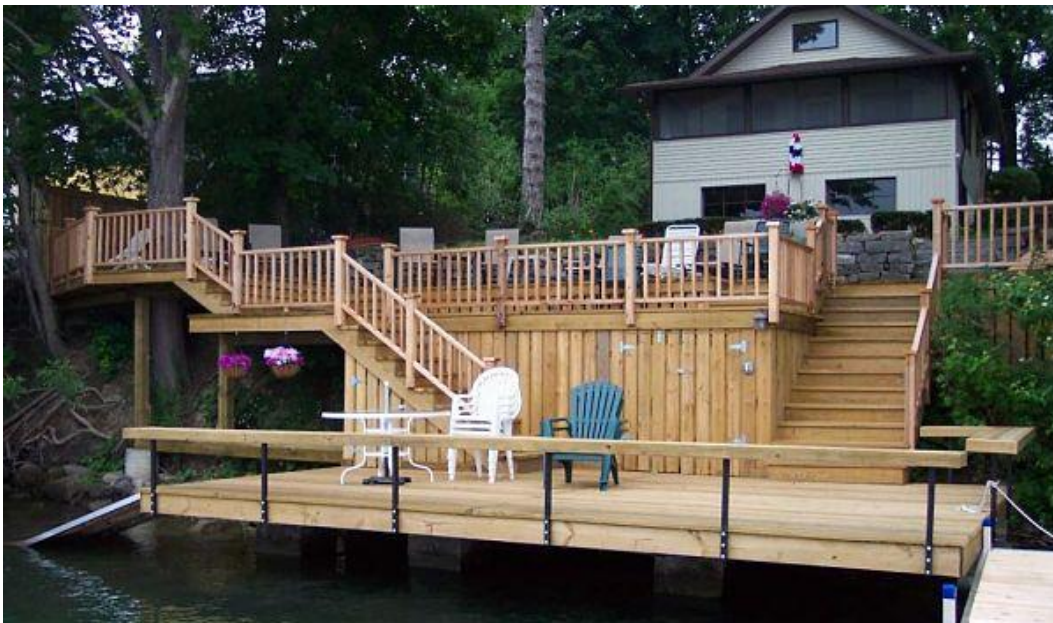
This deck over the water includes concealed storage areas, a ramp into the water, an attached dock and a cutout for an existing tree. Benches incorporated into the deck design provide plenty of seating.
